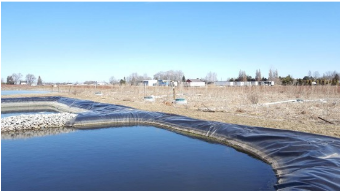
Figure 3.4 Settling Ponds and Constructed Wetland
