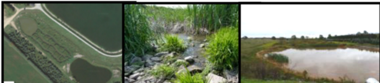
Figure 4.14 Surface flow constructed wetland (aerial view, flow path, and collection pond)
