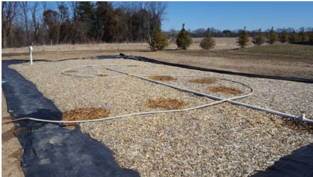
Figure 3.3 Woodchip Denitrification Bioreactor
