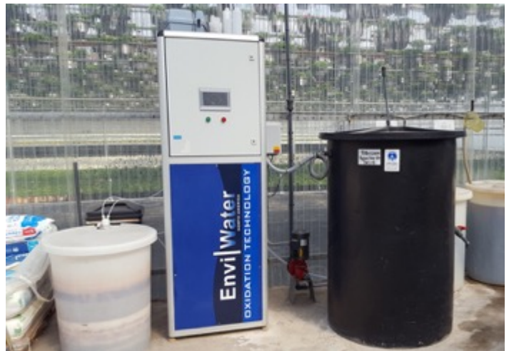
Figure 4.8 Electro-chemical-activation (ECA) system
