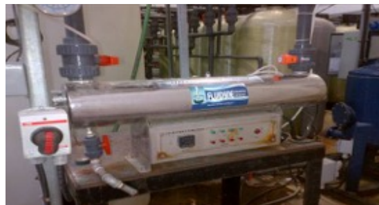
Figure 4.6 Ultra violet treatment systems
