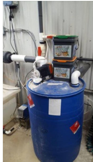
Figure 4.7 ClO 2 injector system
