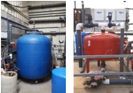
Figure 4.4 Rapid sand filters at two commercial greenhouse operations
