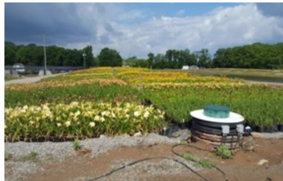
Figure 4.22 Completed HTS with nursery crop production on surface
