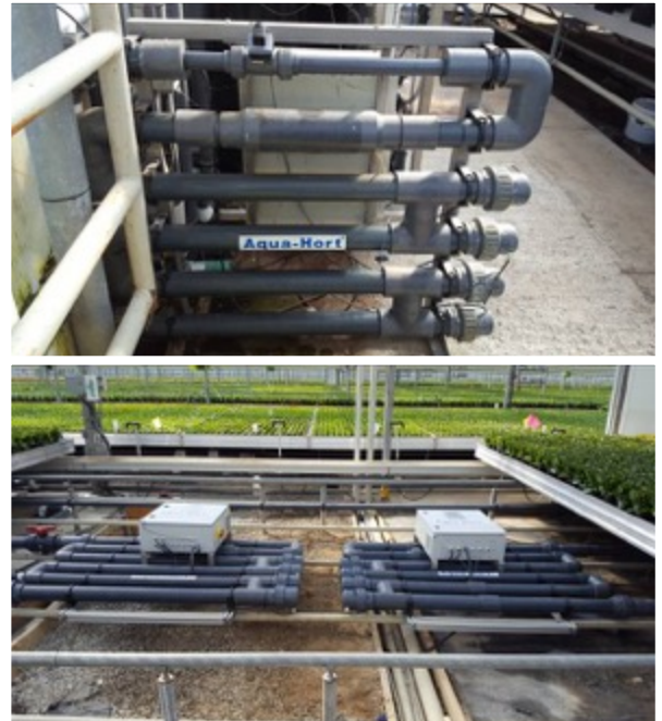
Figure 4.11: Copper ionization systems (Aqua-Hort), vertical and horizontal under bench installations
