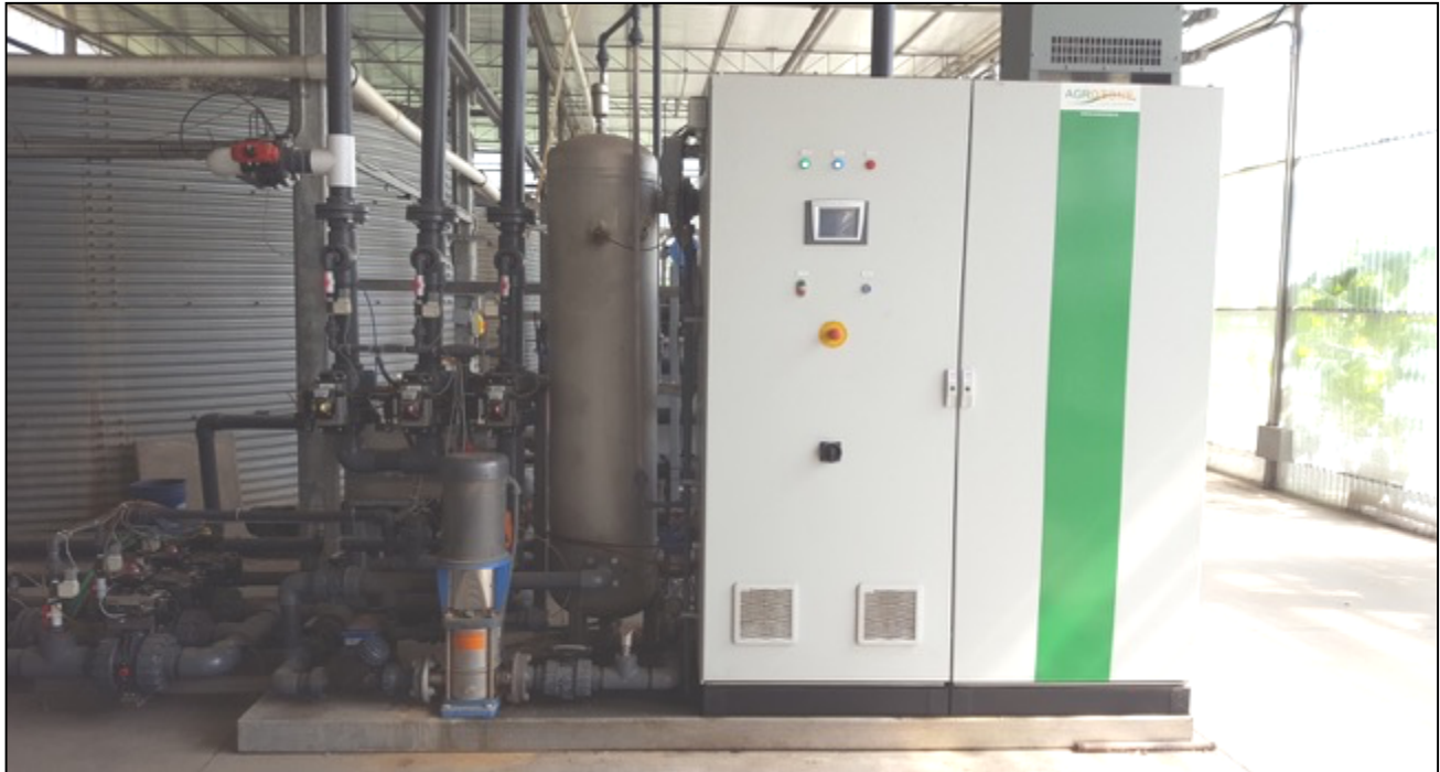
Figure 4.10 Ozone system installed at a vegetable greenhouse
